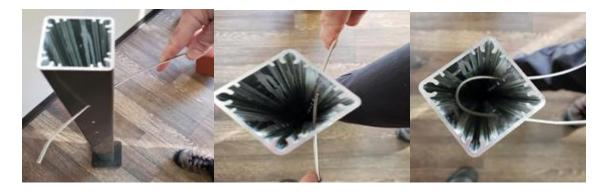
Drop the ½ galvanized pipe into the post through the cable loops. Once the galvanized pipe is all the way in the post, pull the cables towards you to tighten the hold with the pipe. Do this for all cables in the corner post.
