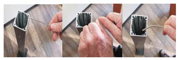
Start by inserting the bent cable through the drilled hole in the post. Then, lace the cable through the post to the corresponding drilled hole on the other side of the post. Do this for all cables. Once the cables are installed through corner post, push the cable back into post to create a loop.
