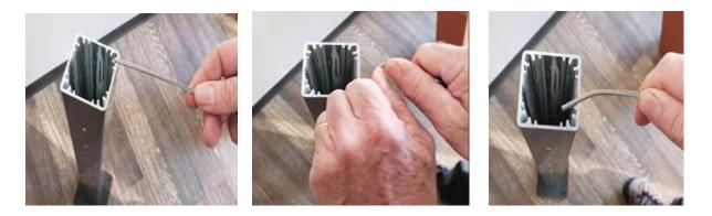
Start by inserting the bent cable through the drilled hole in the post. Then, lace the cable through the post to the corresponding drilled hole on the other side of the post. Do this for all cables. Once the cables are installed through corner post, push the cable back into post to create a loop.
