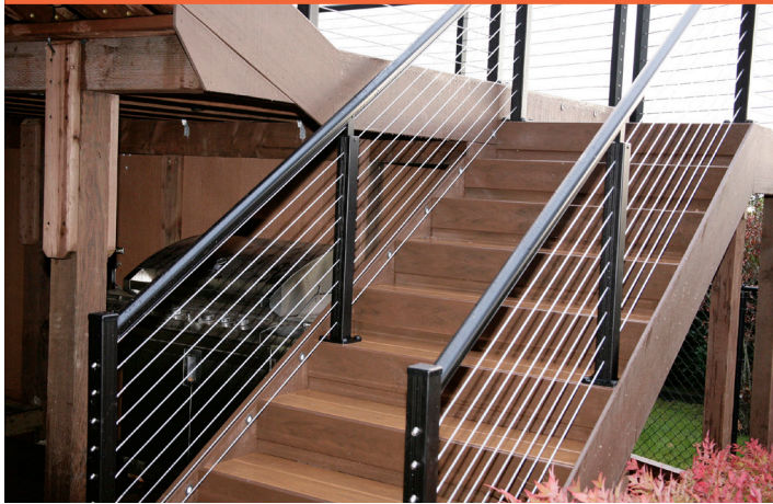
RFX 100 Top Rail over the post using RFX OPF Fitting
